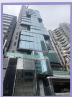
Tsim Sha Tsui New Commercial Building ELV 尖沙咀新商廈ELV項目
