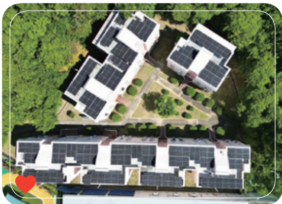
Solar Panels at Staff Quarters in Discovery Bay 愉景灣員工宿舍的太陽能板
