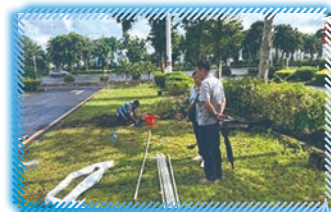
Renovation of reclaimed water pipes in green areas 綠化區域中水管道改造
